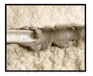
At this point, it is necessary to recognize the fact that a 3/8" masonry joint represents up to 18% of what the eye sees after completion. If you appreciate the stone selection and want to focus on the natural beauty of "all natural thin stone" we recommend narrow grout joints that are raked or recessed back. This will allow the stone to stand out with its natural beauty.
